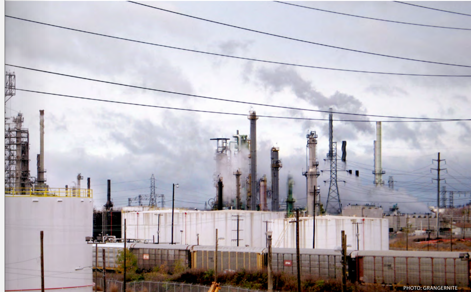
Detroit oil refinery
